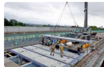
橋梁の床版取替
